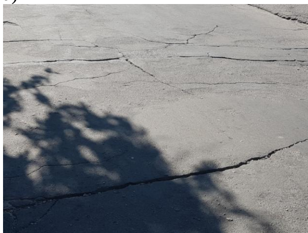
Figure 5 - Cracked asphalt pavement on the Sirko, 47 str. (a) and the position of observation points on a satellite map (b)
