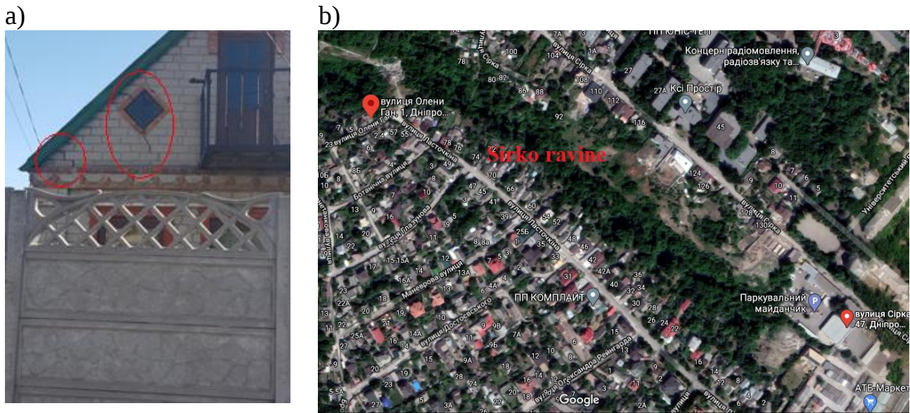
Figure 6 - Deformations of the walls of the house (a) and the position of observation points on the satellite map (b)
